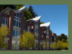
The C. K. Choi Building in Vancouver does not have any air conditioning system within the building. Raised roof monitors are present to draw air in through the vents below and allow stack ventilation to occur. The stack effect induced by the pressure difference present at the lower and upper outlet areas extracts hot air out of the building, thus lowering indoor dry bulb temperature.
